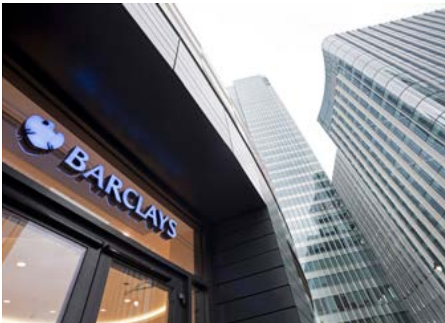
Headquarters of Barclays Bank in Canary Wharf
